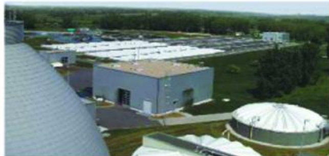
wastewater treatment plant “废水处理厂”
